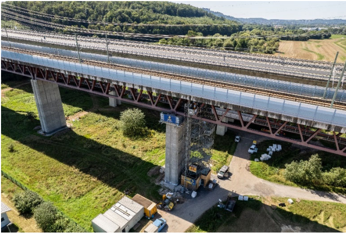
(3) Work on the pier caps was executed using suspended scaffolding.
