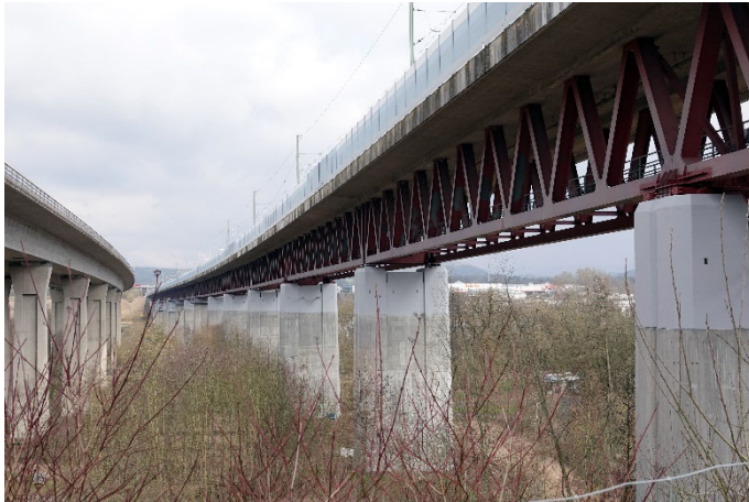
(6) The freshly renovated pier caps of the Itztal bridge railway overpass
