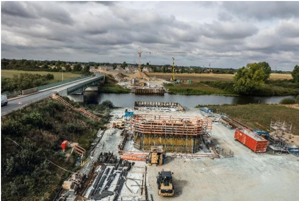
(3) Bored pile foundations were installed for the bridge piers.
